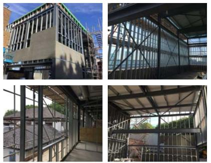
Base / head channel to concrete Vertical rail to head track and base track Sheathing boards to light steel frame Sheathing boards to aluminium Sheathing boards to timber frame
